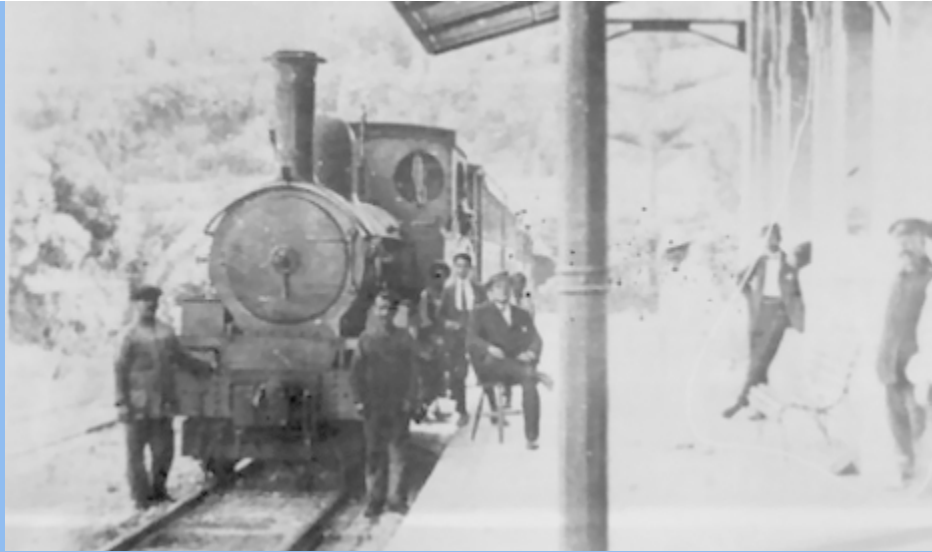
Trams disappeared from Malta in 1930's - Photo Malta Transport Authority
